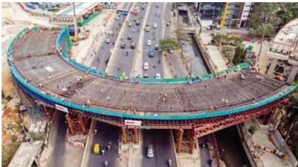
Solid slab running 125 metre cast by BMRCL at Central Silk Board(Photo | Express)
