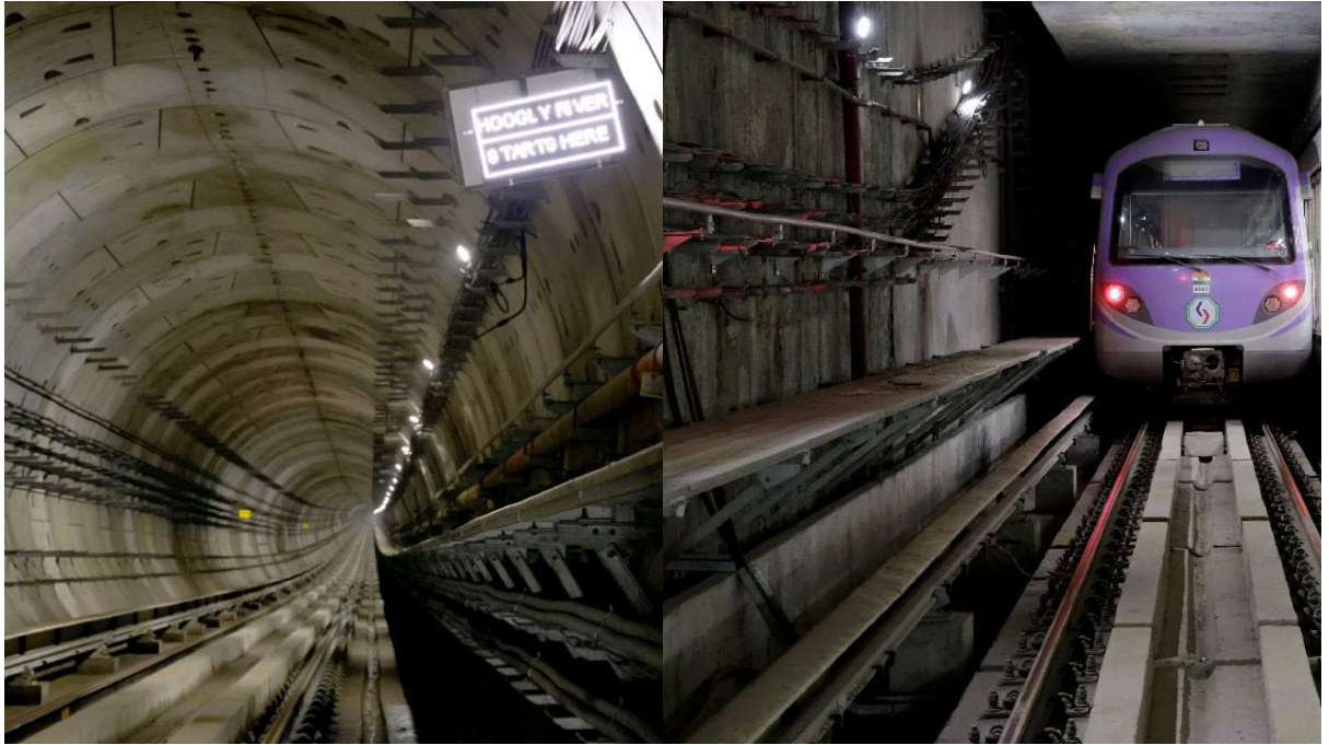
India's first underwater metro line, will begin operations from March 15 Follow us
