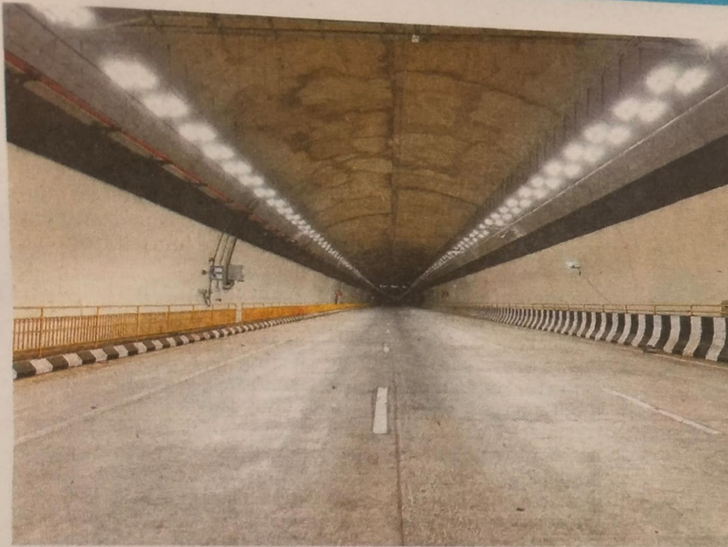
The 7.78 km wide twin tunnels running through the Igatpuri – Kasara Ghat section is widest tunnel in India with a width of 17.6 metres.
