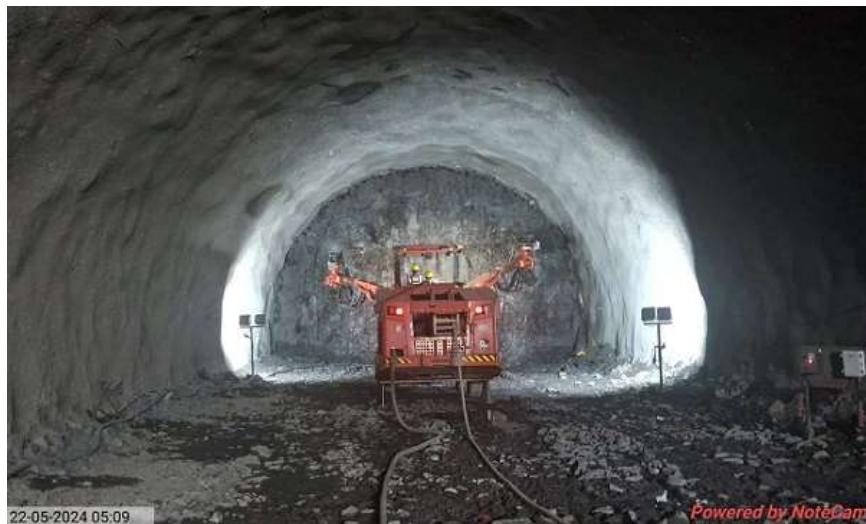
The ADIT tunnel's portal is located at Ghansoli, Navi Mumbai (view on [Google Maps](#)). From its extreme-end, NATM tunneling will be done towards opposite sides – westward to Sawli's Shaft-3 for 1.6 kms and eastwards towards Shilphata's tunnel portal covering a distance of roughly 1.8 kms.
