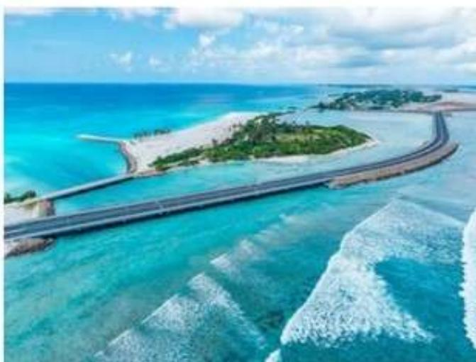
In Addu City, Afcons has completed the Addu City Development Project which includes 111 km of roads, a detour link road of 1.4km consisting of two ocean bridges, 106 km of drainage works, 160 km of Street Lighting, 376 CCTV Cameras, 41 km of Utility Duct and 38 pumping stations across Hithadhoo, Maradhoo, Maradhoo-Feydhoo, Feydhoo, Hulhudhoo and Meedhoo. It has significantly improved mobility, public safety and brought relief to residents from frequent flooding among others.
