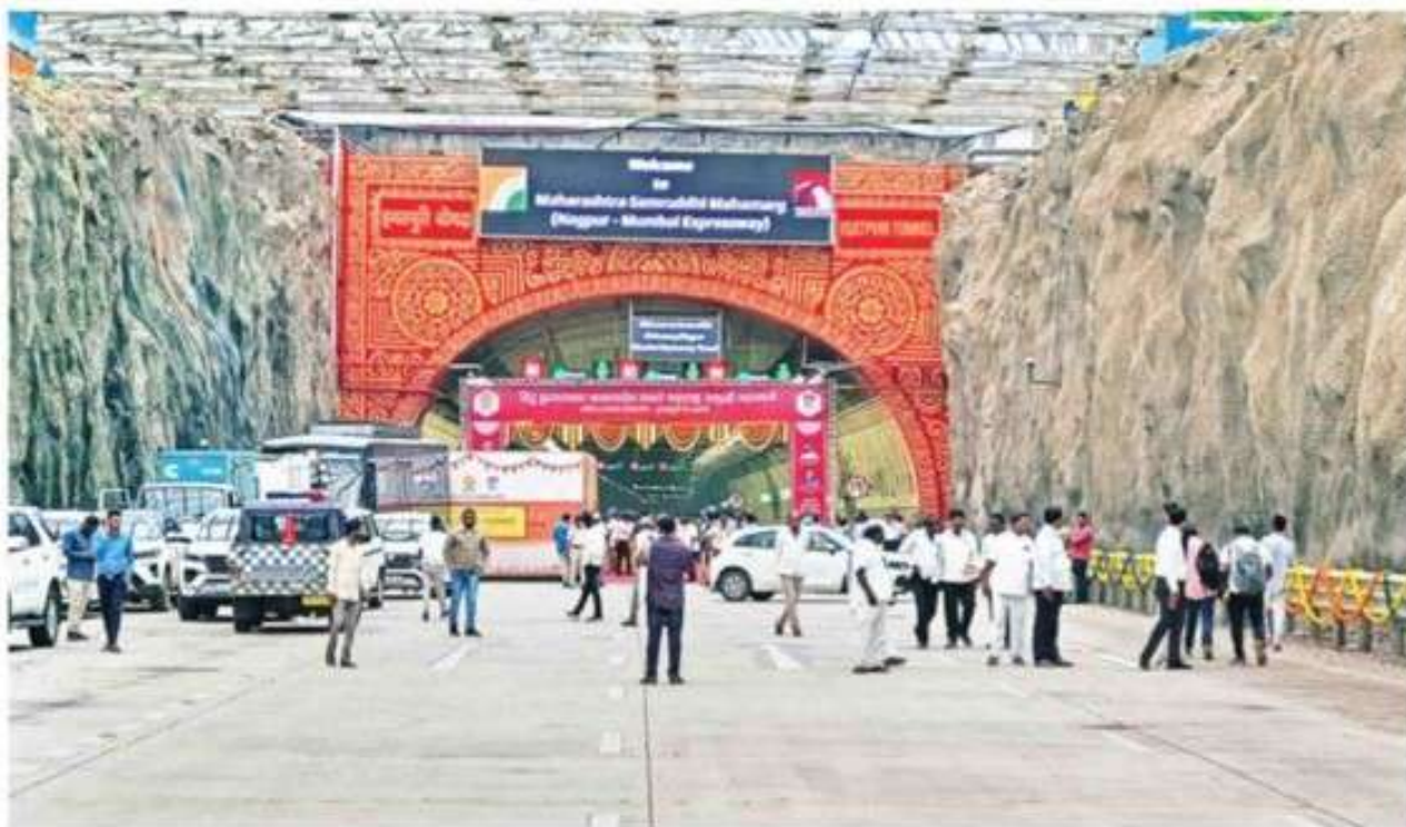
India's widest tunnel that is part of the Mumbai-Nagpur Samruddhi Mahamarg that was opened fully on Thursday. Deepak Joshi
