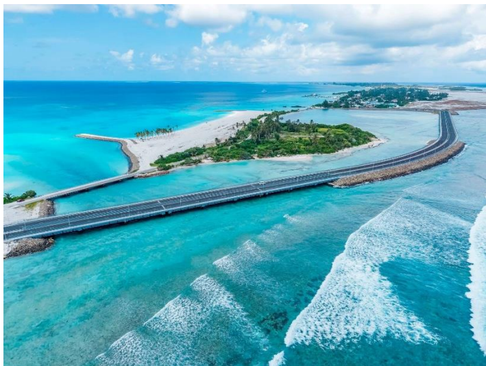
A detour link of 1.4km, Addu City Development Project
