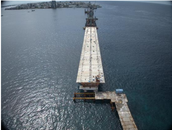
Erection of segments being carried out in Greater Male Connectivity Project, Maldives
