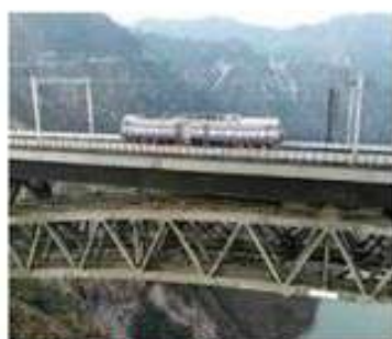
CHENAB BRIDGE. Engineering marvel on
