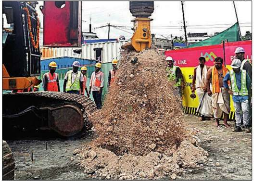
Inauguration of Kochi Metro Phase II works held at Kakkanad on Wednesday
