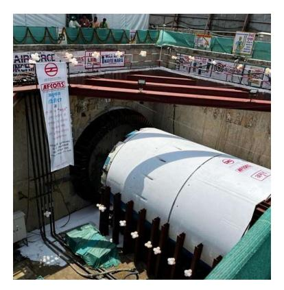
In the coming days, TBM Amrit's cradle will be pushed to make Amrit's cutterhead align with the head-wall's eye seal. Installation of temporary rings within the shaft and initial drive will follow.
