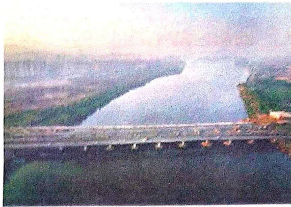
The Kasheli creek bridge consists of 13 spans, including nine over water
