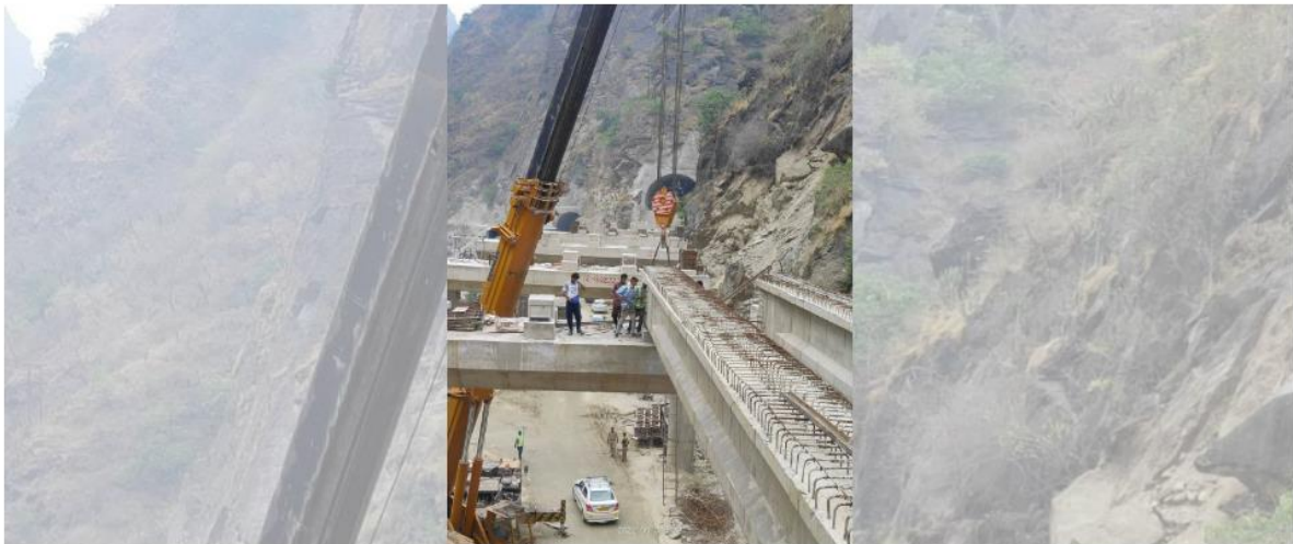
Work in progress on Chandigarh-Manali highway near Takoli.
