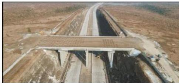
A view of the wildlife pass constructed on Samruddhi Mahamarg in Wardha district.
