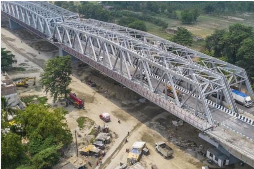
Almost 66,360 metric tonnes of steel have been used in the entire bridge superstructure. Pic/News18
