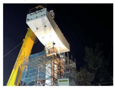
KANPUR: UP Metro Corporation Limited successfully placed the first 'Cross Arm' at IIT-Kanpur Station under the Priority Corridor, being constructed between IIT-K and Motijheel. In future, it will be used to extend the length of the metro stations.
