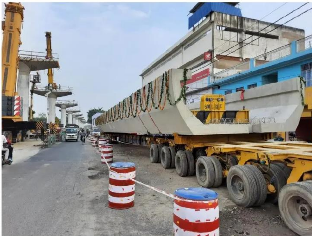
The U Girders being erected.
