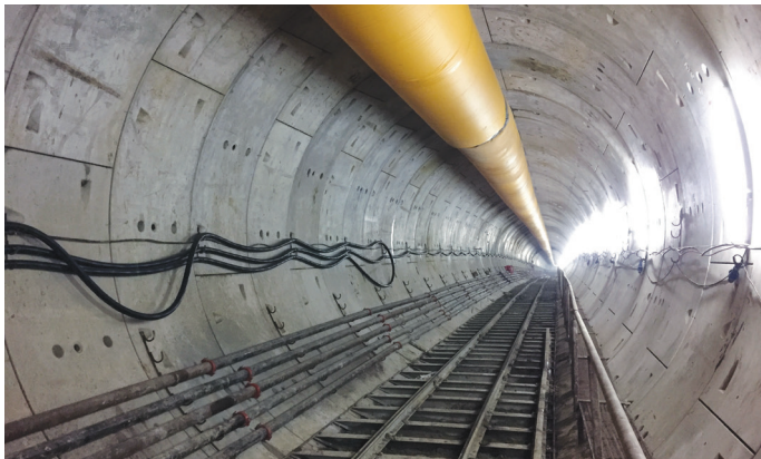
Afcons has completed construction of India's first twin underwater Metro tunnels, in Kolkata, for the East West Metro Project. The tunnels are at a depth of 32m below river Ganges
