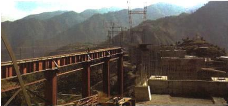
View of the ropeway pylons from a fabrication yard
