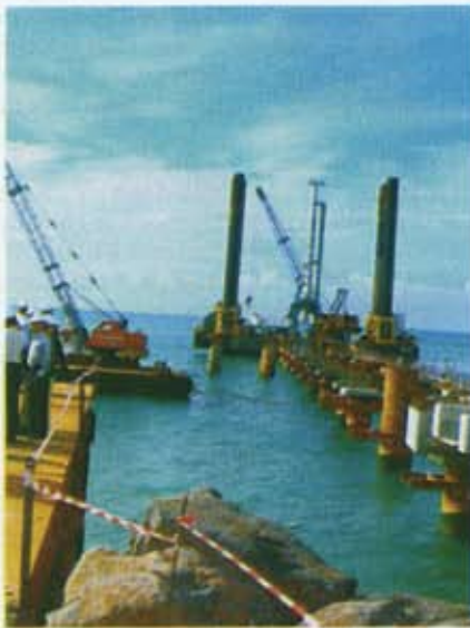
Oil jetty project in Mauritius
